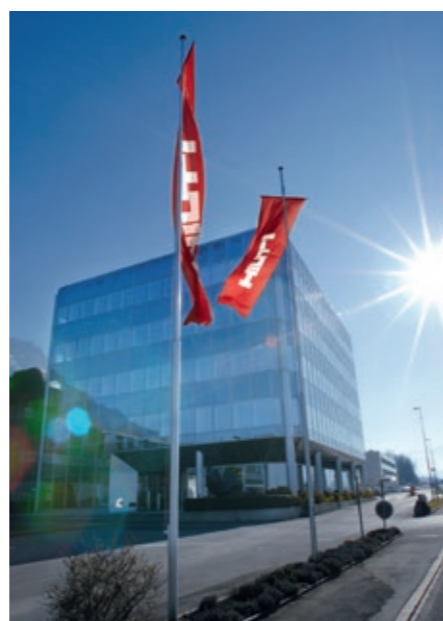
The main administration building at Hilti corporate headquarters in Schaan, Liechtenstein.
